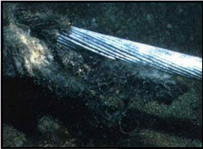
Cable damaged by trawling gear
