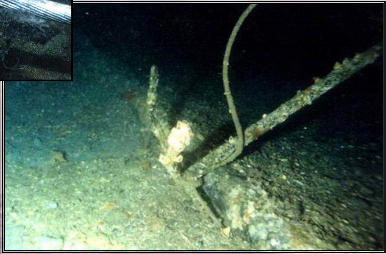
Cable snagged & moved by trawling gear Courtesy: Seaworks & Transpower NZ
