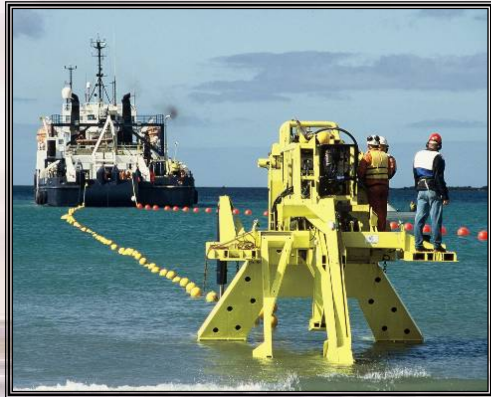
Sea plough & cable ship about to bury cable Courtesy: Seaworks, NZ
